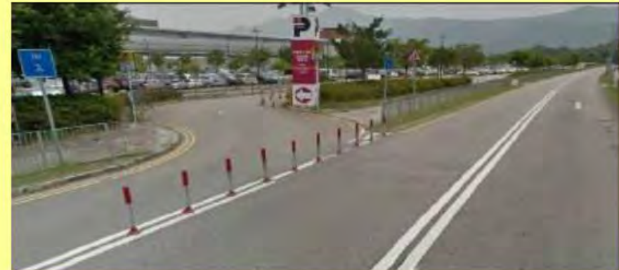
Kam Sheung Road Station
