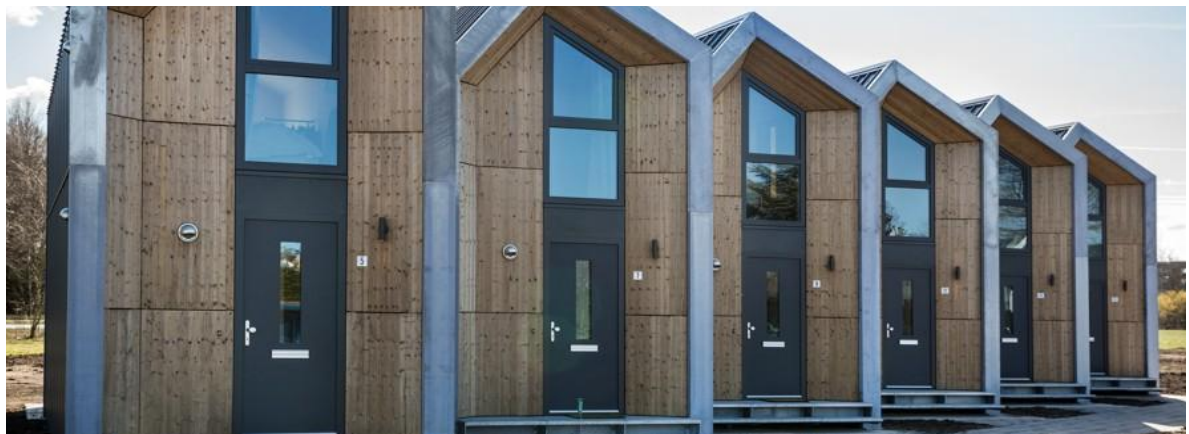
Illustration: The Heijmans One "Tiny House" prototype has been installed at sites across The Netherlands.
